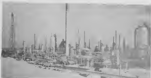
The hydrodesulfurization complex
